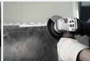
Removing welded seams
